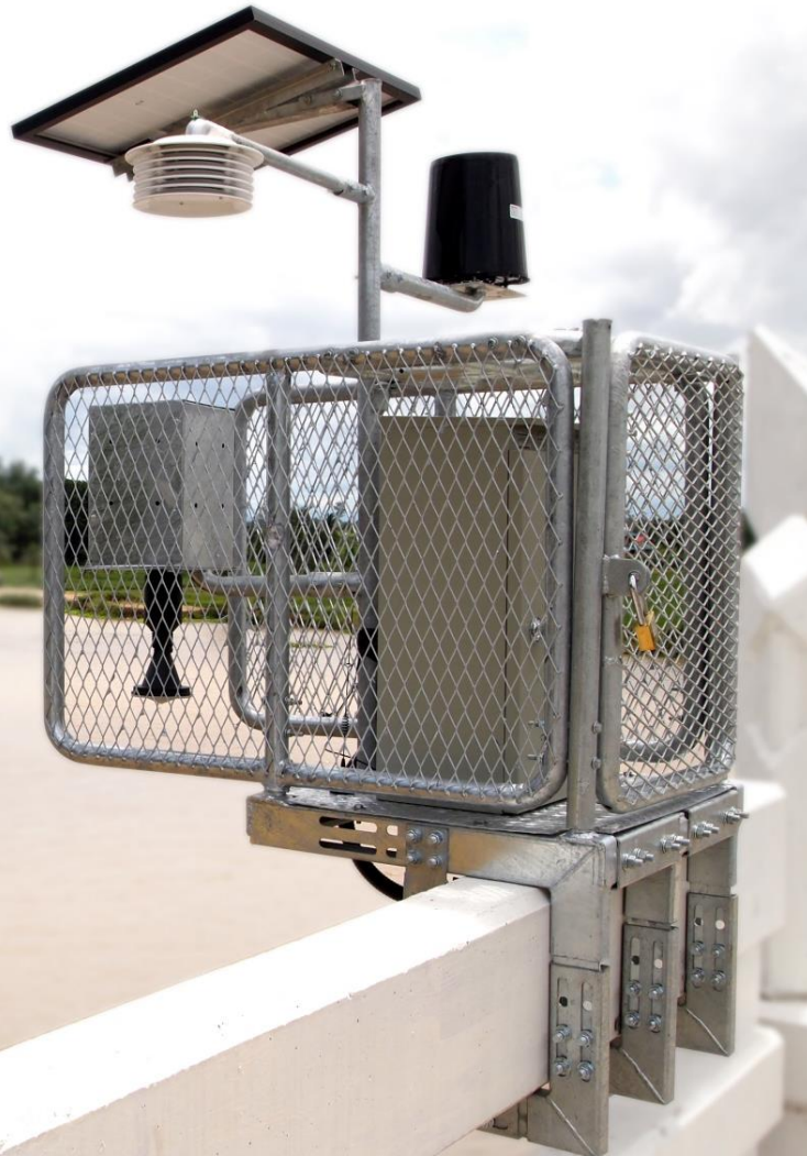
Weather + Water Level Telemetry Station
